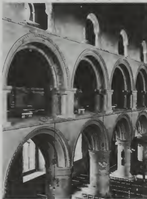
Romanesque archivolt over the arches of the nave of Southwell Minster, Nottinghamshire, England, mid-12th century
